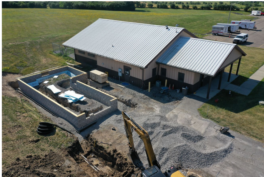
Photo: Aerial view of Livingston County Dog Control expansion underway
